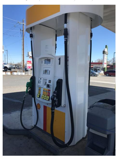
Photograph 2 Date: 03/31/2021 Photo illustrating new dispenser and a Balance Vapor Recovery nozzle. **Direction:** E
